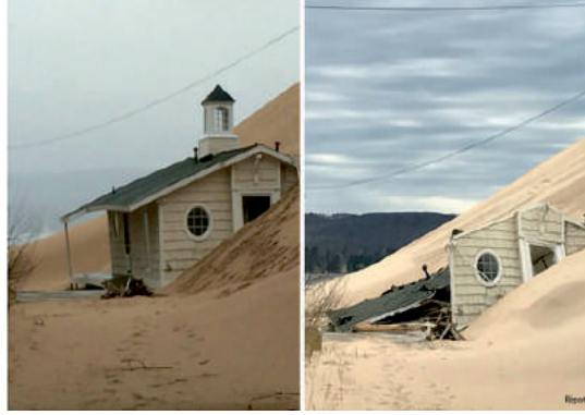
Figure 5.3: Sand Ultimate Limit States. House collapse due to active lateral sand pressure from an encroaching sand dune at the Silver Lake in Michigan, before and after the attainment of the SULS.
