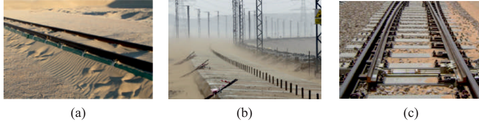
Figure 2.33: Sand-resistant Receiver SMMs. Ballastless track slab systems: longitudinal continuous support, T-Track system (a, explicit publishing permission from the owner of the photo: Giles Wiggs), continuous slab (b, reprinted from [200], with the permission from El Confidencial). Lubricant free turnout (c, reprinted from [154], with the permission from Voestalpine).
