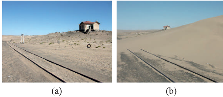
Figure 2.10: Grasplatz railway station along the Aus to Lüderitz railway before (a) and after (b) sand dune encroaching (permission to reuse under a Creative Commons Attribution License; owner of the photo: [68]).
