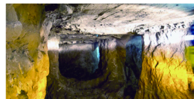
Fig. 15. Quarry site analyzed and the room-pillars system is clearly noticeable.
