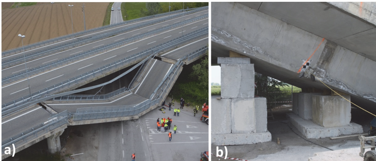
Figure 7: Overview of the collapsed Fossano bridge (a) and structural scheme (b).
