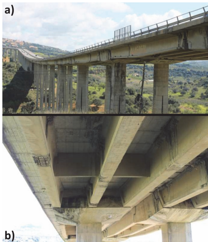
Figure 13: Overall view of the Akragas viaduct (a); deck detail (b) [23].
