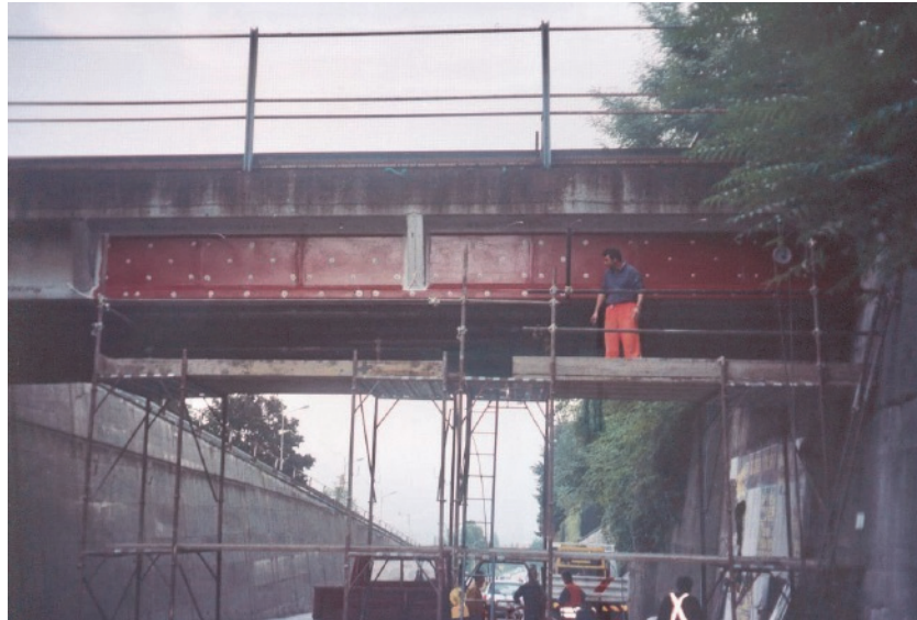
Figure 19: Steel resurfacing for I-beams of an overpass [Copyright: RELUIS].
