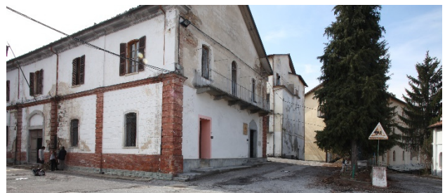
Figure 2. A view of a part of the Giuseppe Galliano Barrack in Mondovì.
