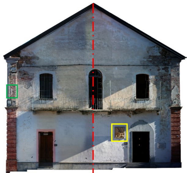
Figure 5. Orthophoto of the north façade generated using Pix4D (left) and MicMac (right)
