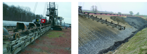
(a) Chain bucket excavator operating onsite, front view (b) Chain bucket excavator in operation in silty soil, lateral view
