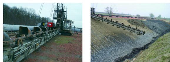
(a) Chain bucket excavator operating onsite, front view
