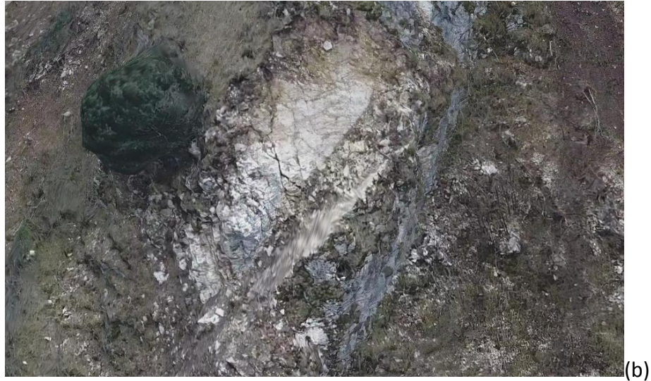
Figure 4.63. General oblique view of the rock slide and subsequent rock avalanche on the left flank of the Nera valley (km 3 of SP134 motorway) (a); detail of the detachment area (b). Images taken from the 3D model generated by BYU on the basis of drone surveys.
