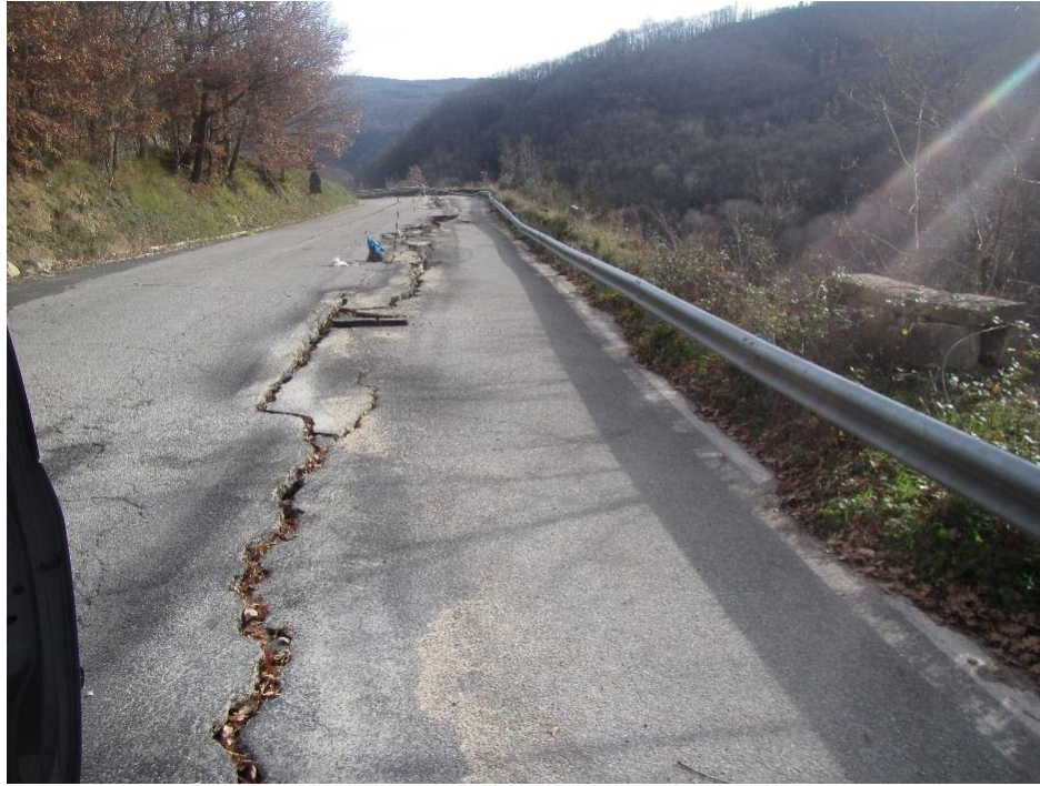
Figure 4.17. Road damage induced by slight rotation of the underlying retaining wall and/or settlement of the retaining wall backfill.
