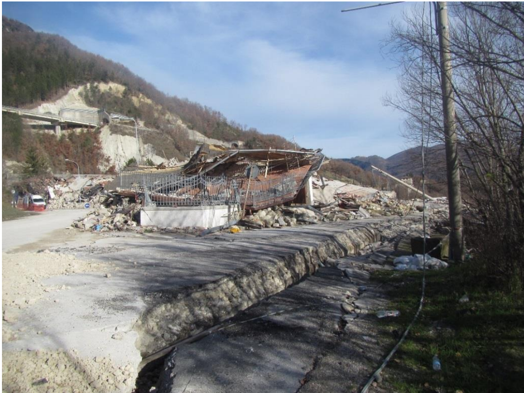
Figure 4.16. Pavement and road base damage induced by underlying stability failure of fill material (Location 3c).
