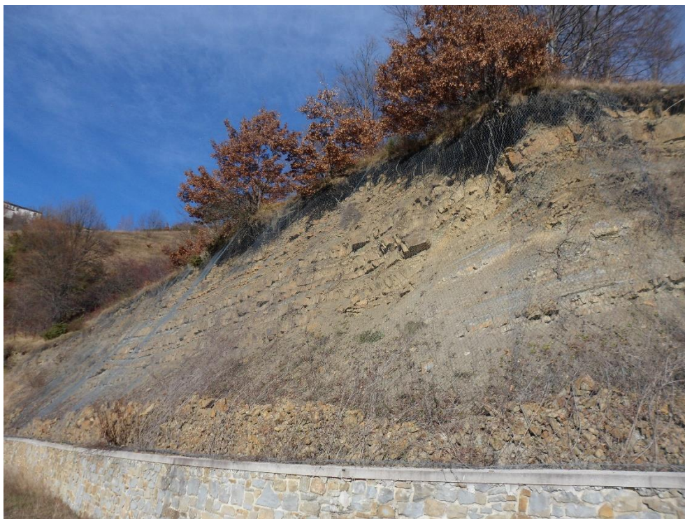
Figure 4.97. Rock-net protection with captured debris.
