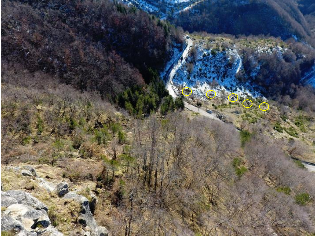
Figure 4.51. UAV image of rockfall site near Crognaleto village from the source area at the top of slope looking down to road along runout chute. Note several large 1 to 3 meter boulder fragments in the drainage below the road (yellow circles).
