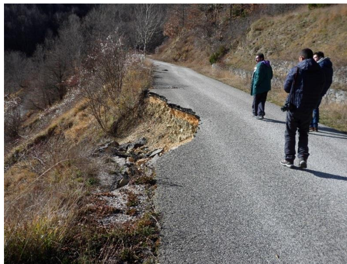
Figure 4.93. A slide observed on the fill slope.
