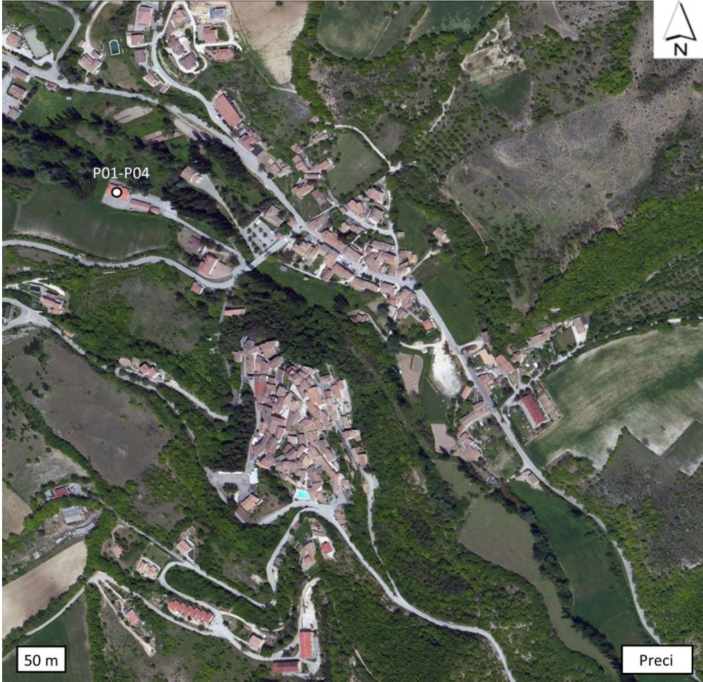
Figure 6.110. Locations of the representative structures inspected in Preci.
