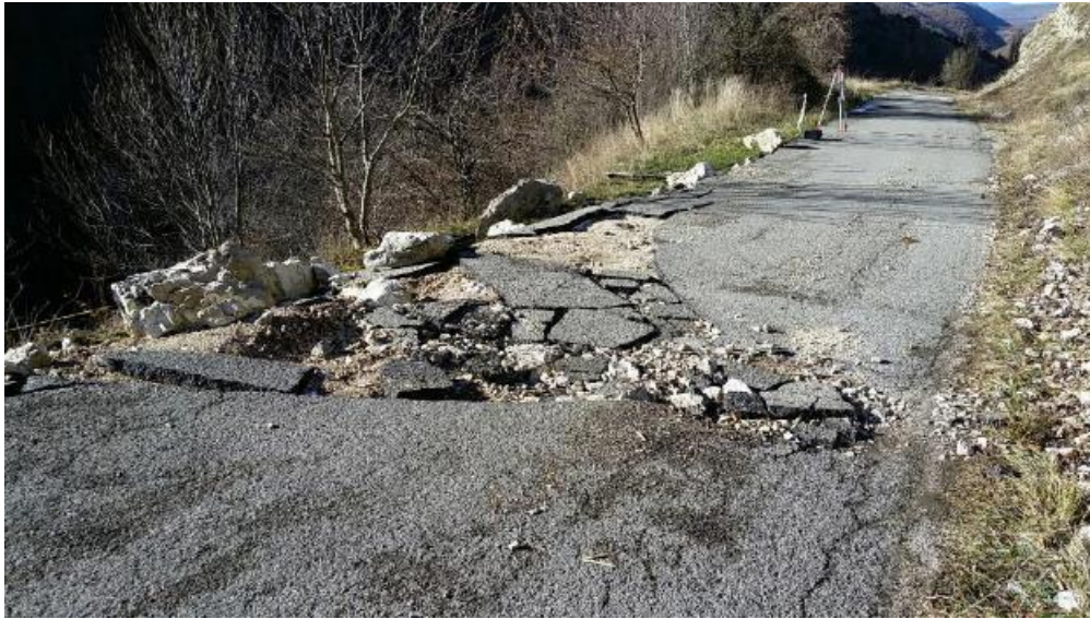
Figure 4.58. Damage to road from 1-2.5 m boulder impacts from rockfall between sites 9a and 9b.
