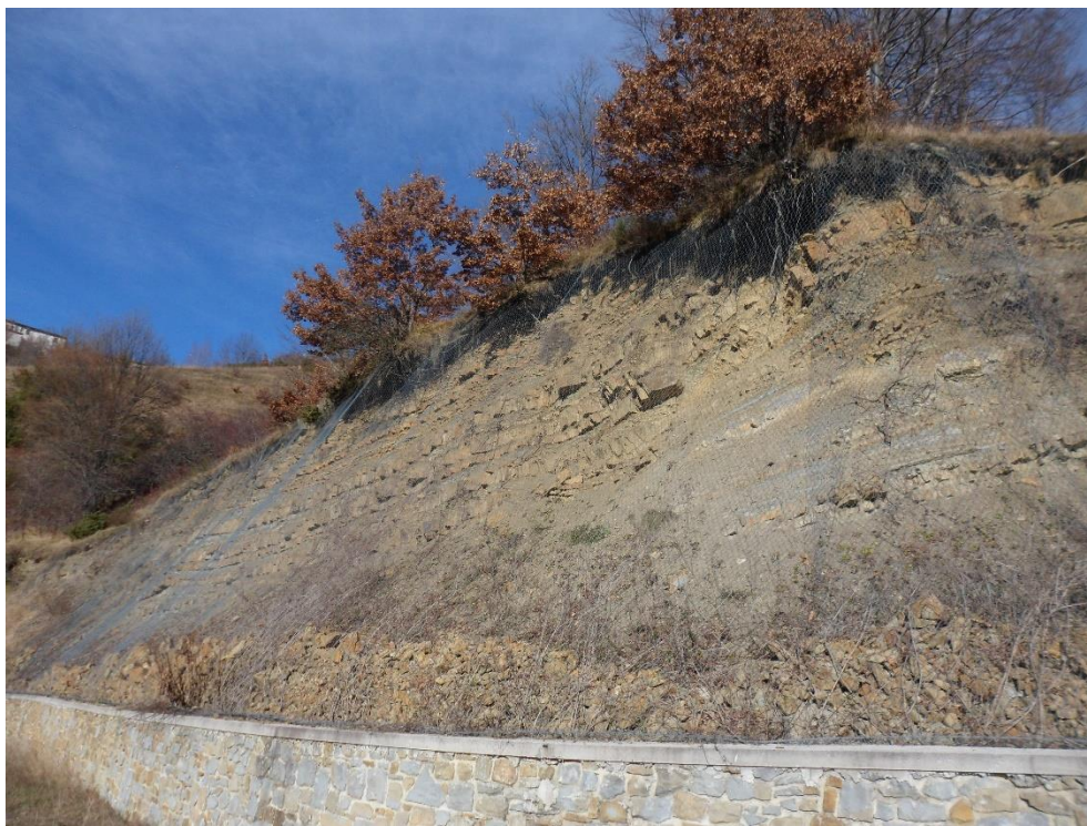
Figure 4.97. Rock-net protection with captured debris.
