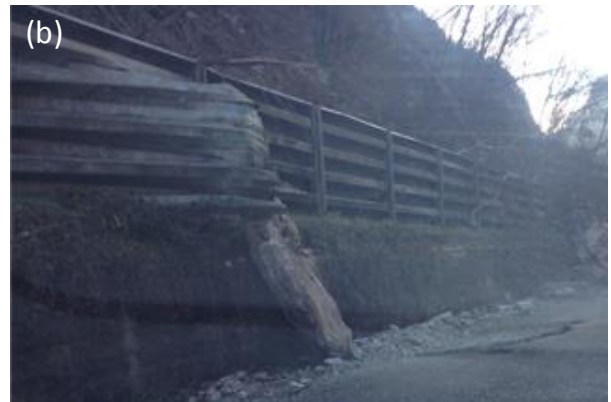
Figure 4.82. Rockfalls along the SP209 between Triponzi and Visso.
