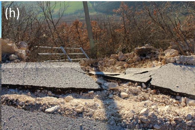
Figure 4.79. Fracture along the road, large vertical offset due to fracture and ultimate movement, damaged edge barriers and debris and boulders on the road surface.
