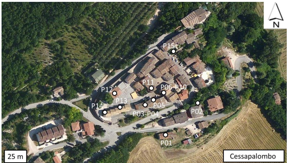
Figure 6.108. Locations of the representative structures inspected in Cessapalombo (see Table 6.17 for details).
