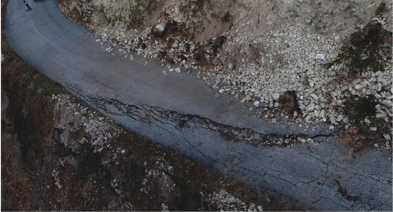
Figure 4.39. 3D model of the western half of the Valle di Panico landslide headscarp.
