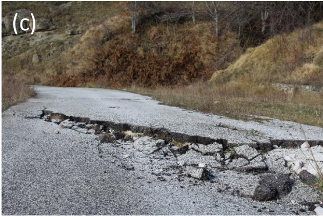
Figure 4.92. Cracks along the road.
