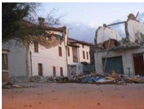
Figure 6.128. Pictures of the structures with assigned damage level D5 in San Pellegrino, before and after the October earthquake, along with their identification numbers.
