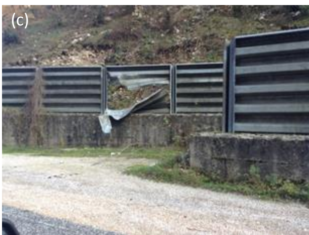
Figure 4.83. Slope protection damaged by boulders and rock-blocks.
