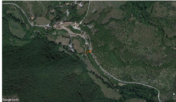
Figure 4.98. Location of the rockfalls along SP476 (between Piedivalle and Preci).
