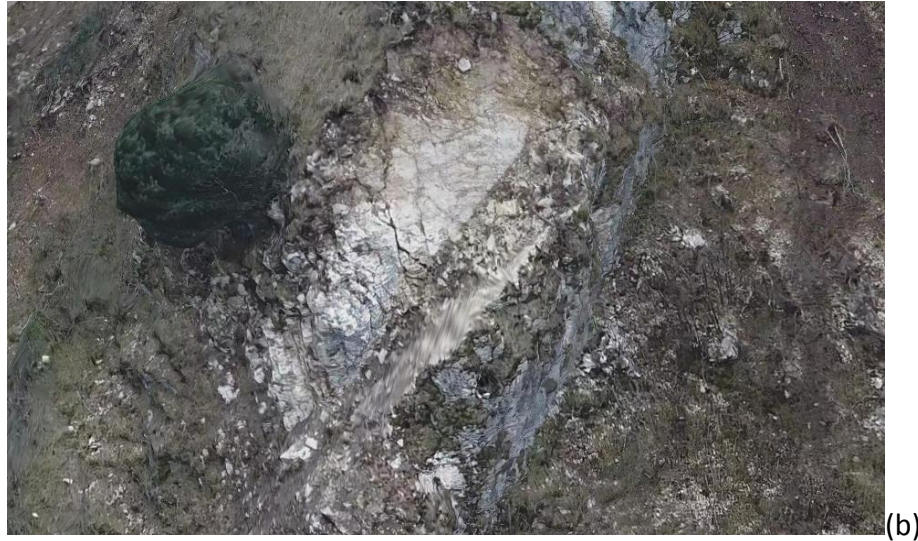
Figure 4.63. General oblique view of the rock slide and subsequent rock avalanche on the left flank of the Nera valley (km 3 of SP134 motorway) (a); detail of the detachment area (b). Images taken from the 3D model generated by BYU on the basis of drone surveys.
