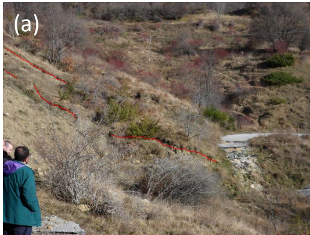
Figure 4.94. Fractures on the cut slope.
