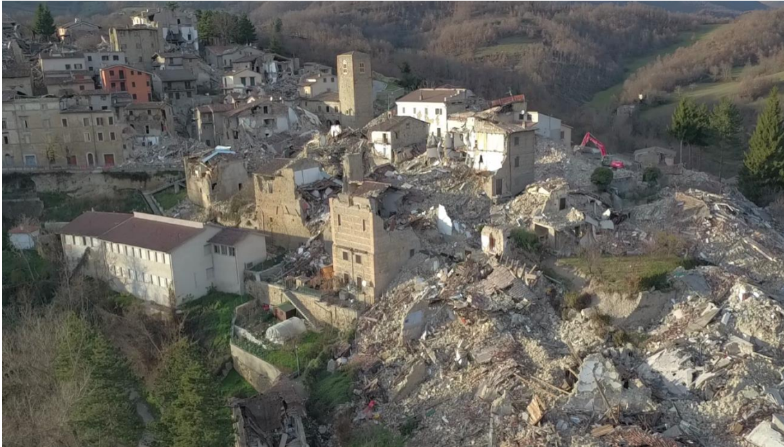
Figure 6.23. Aerial view, south-north direction (V5).
