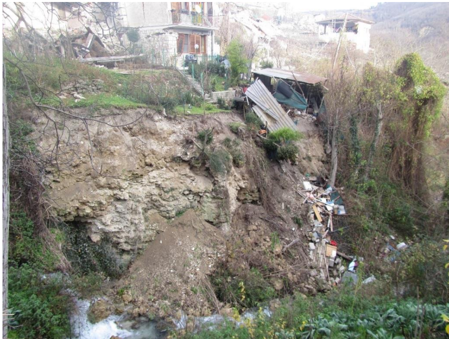
Figure 4.20. Failure of steepened talus gully wall material and crest area above (Location 3e).
