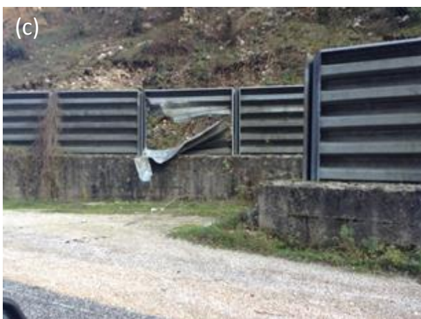
Figure 4.83. Slope protection damaged by boulders and rock-blocks.
