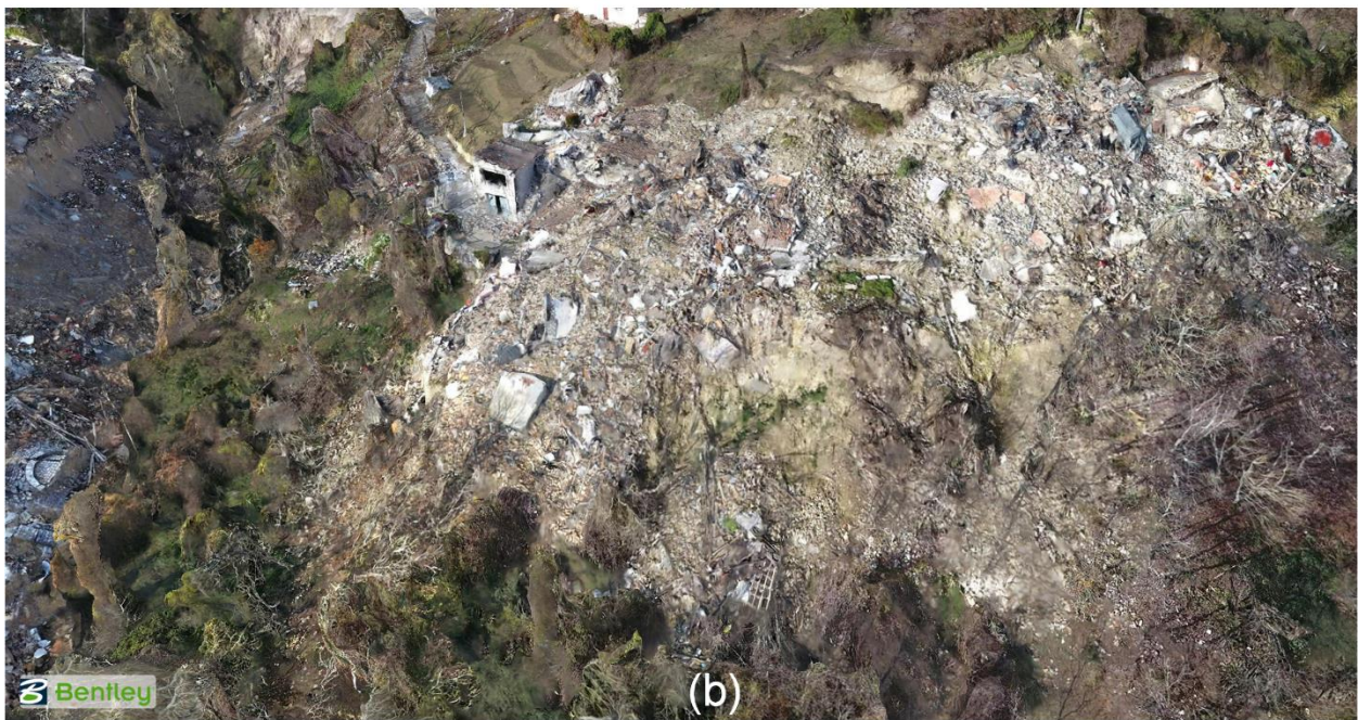
Figure 4.27. 3D model comparison of the landslide beneath the northern slope of Pescara del Tronto between September 2016 (a) and December 2016 (b).
