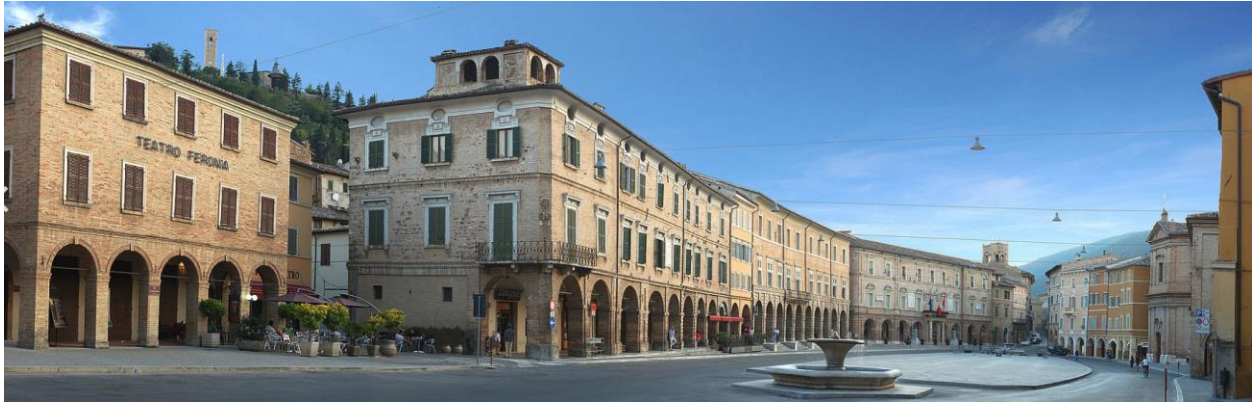
Figure 6.76. Piazza del Popolo, San Severino Marche (before seismic events).
