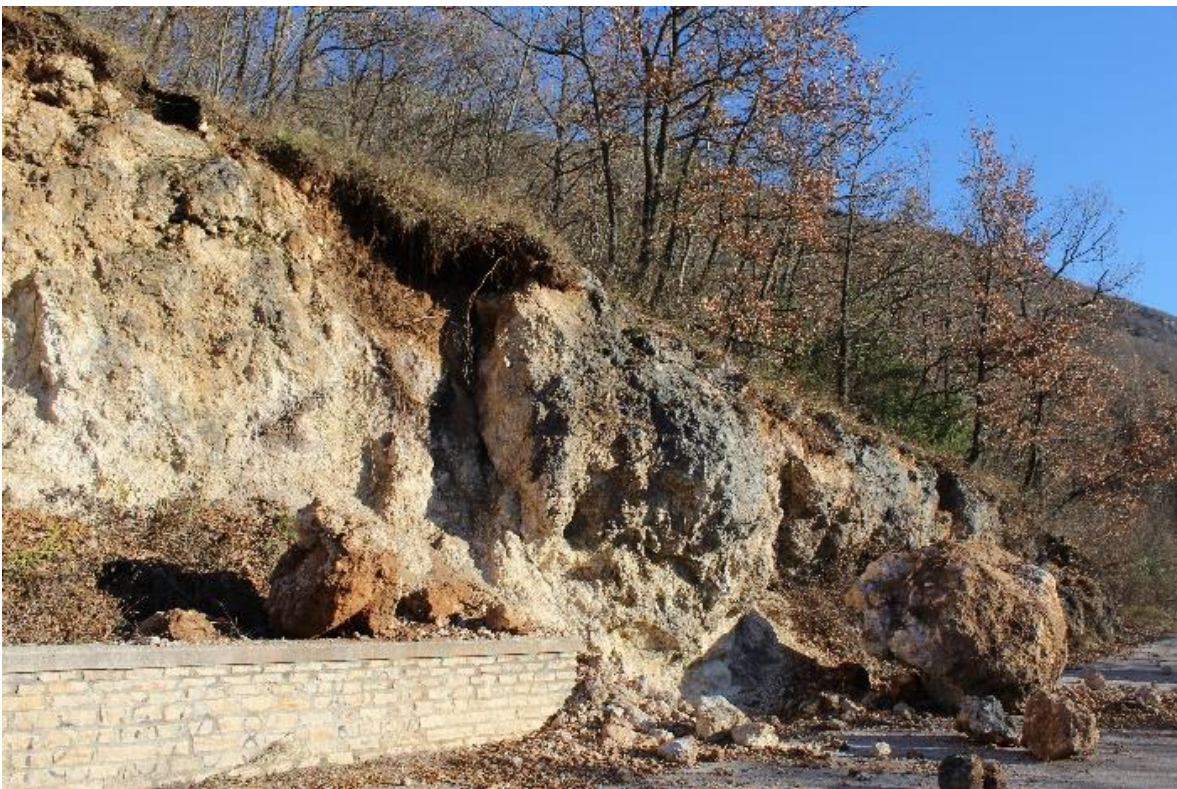
Figure 4.74. Rockfalls with boulders on the road.
