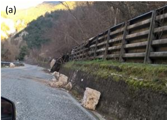
Figure 4.82. Rockfalls along the SP209 between Triponzi and Visso.
