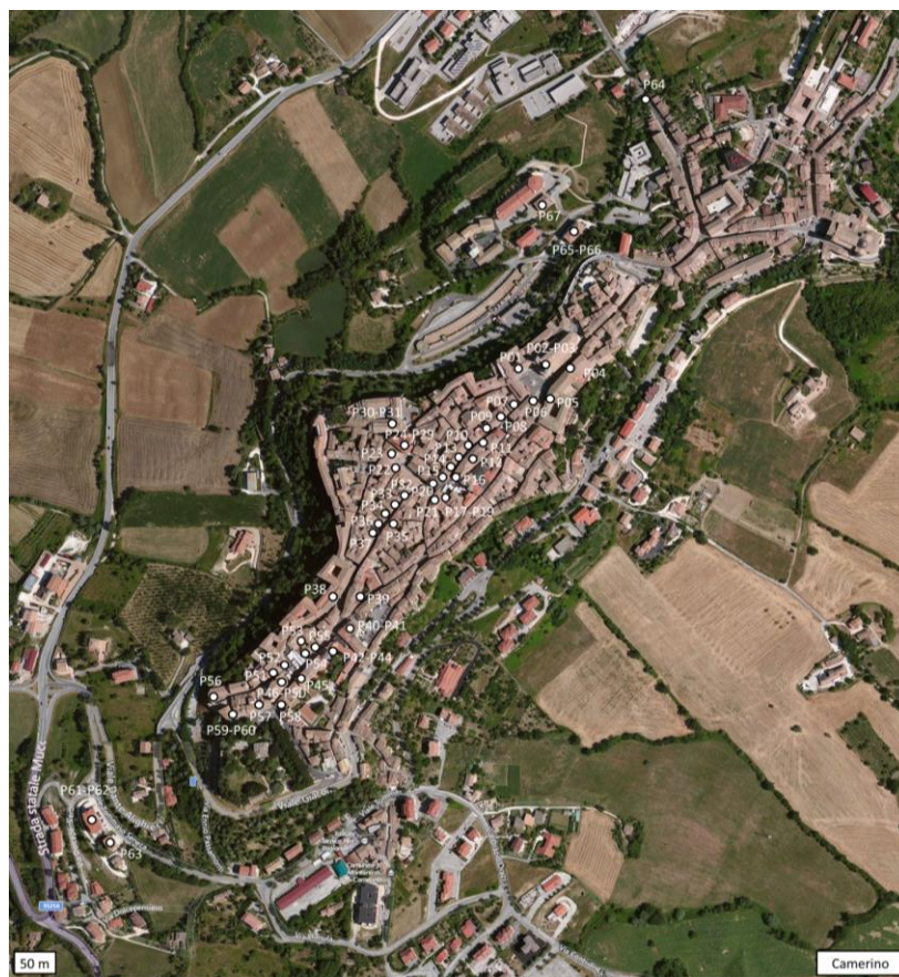
Figure 6.83. Locations of the representative structures inspected in Camerino (including red zone) (see Table 6.11 for details).
