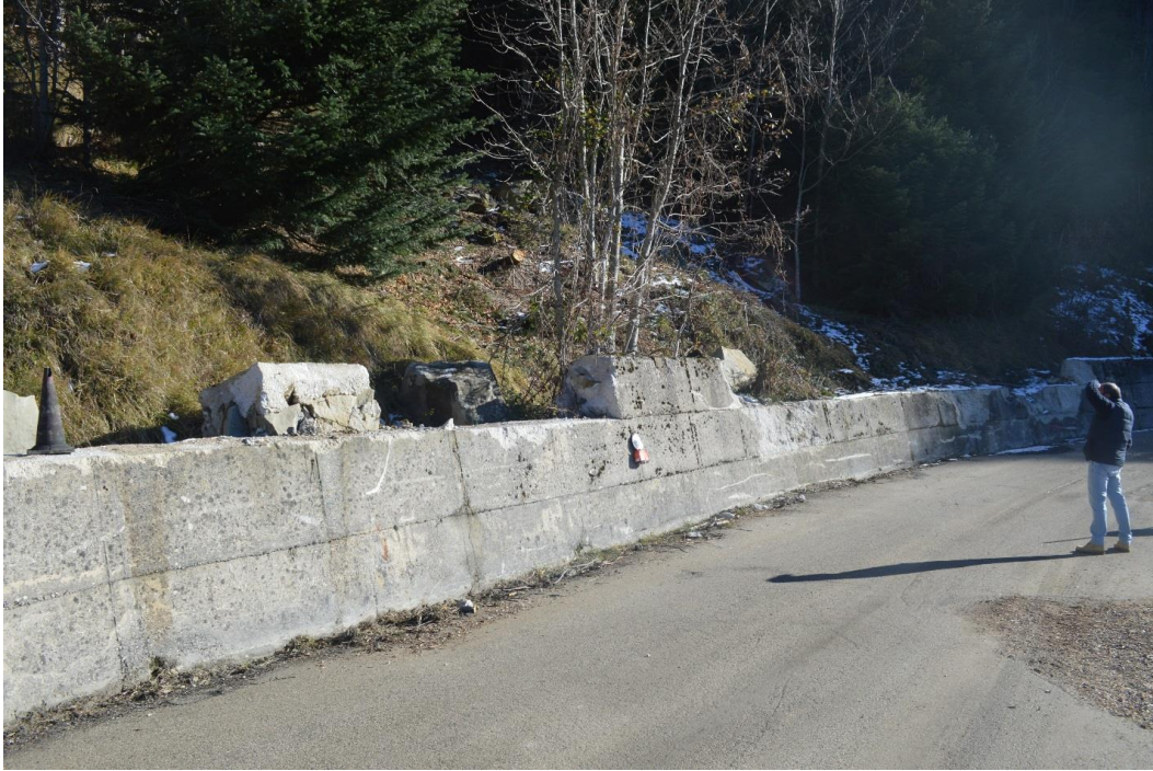
Figure 4.52. Damaged segmented concrete block retaining wall at roadway. Blocks that fell on road have been removed by local officials prior to visit from GEER team.
