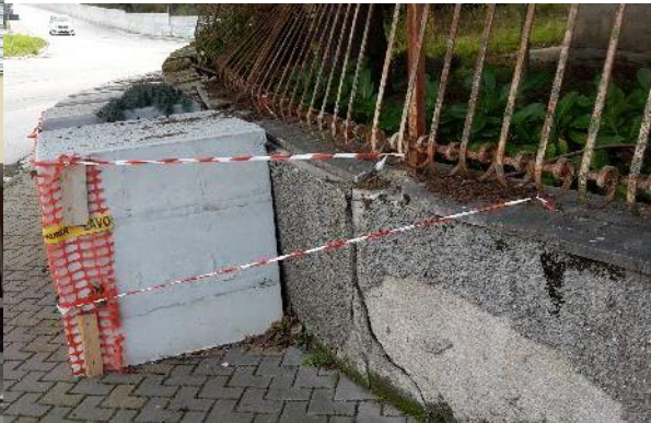
P11 (Retaining wall)
