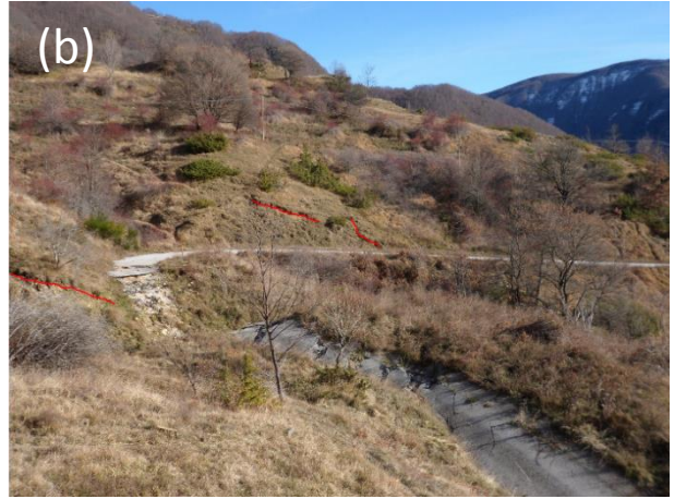
Figure 4.94. Fractures on the cut slope.
