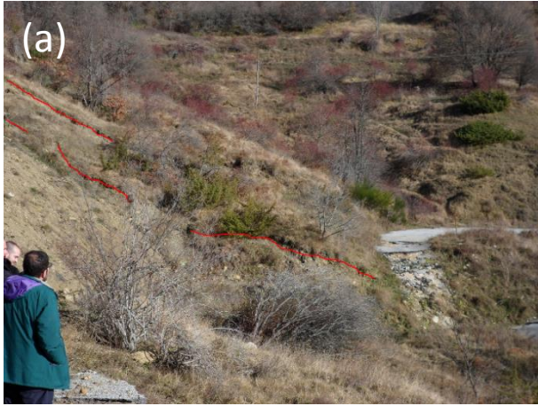
Figure 4.94. Fractures on the cut slope.
