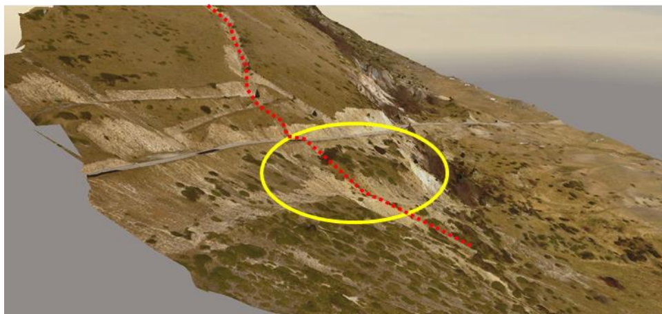
Figure 4.104. 3D SfM model of embankment fill damage area next to fault trace zone along SP477 road, Mt Vettore. Fill that has experienced 15 to 20cm lateral displacement circled in yellow. Observed fault rupture trace shown in red.
