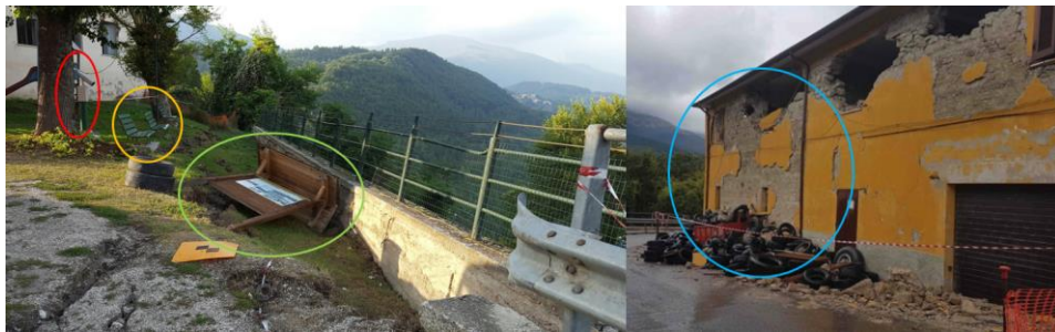
Figure 6.26. Representative pictures of landslide in eastern part of village (September 2016).
