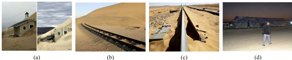
Fig. 6. Windblown Sand Ultimate Limit States. House collapse due to active lateral sand pressure from an encroaching sand dune at the Silver Lake in Michigan, (a), before and after the attainment of the SULs), full sand coverage of a railway due to encroaching sand dune in Namibia (b), explicit publishing permission from the owner of the photo: Giles Wiggs), railroad switch jammed by sedimented sand in Algeria (c), train derailment in Namibia (d, reprinted from [34] with the permission from the editor).
