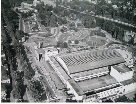
FIGURE 1: Aerial view of the Turin Exhibition Centre: the large hall with the semicircular apse is Hall B built in 1948.
