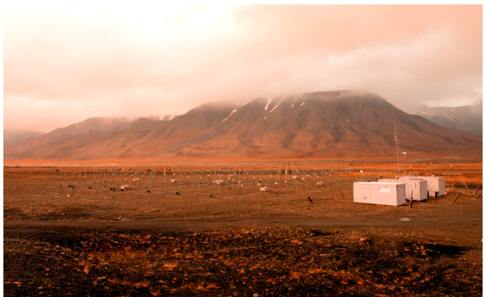
Figure 4. Sousy Radar Station in Adventdalen Valley 78°10'10.05"N, 15°59'33.32"E, Longyearbyen, Spitsbergen (Norway).
