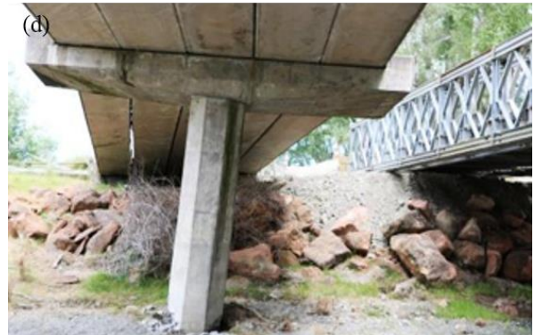
Lower Mason River Bridge; (c) Mason River Bridge; (d) Wandle River Bridge (Palermo et al., 2017).
