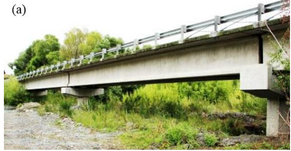
Figure 3. Bridges under study: (a) Lottery River Bridge; (b)
