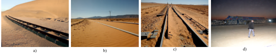
Fig. 2 Sand Ultimate Limit States: full coverage by encroaching sand dune (a, explicit publishing permission from the owner of the photo Giles Wiggs), partial coverage in a sandy plain (b), jammed turnout (c), train derailment (d, reprinted from [6] with the permission from the editor).
