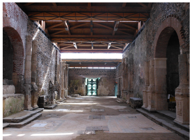
Figure 5. Interior of the church
