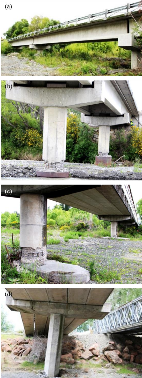
under transverse loading such that they can displace an appreciable amount on the supporting elastomeric bearings before contacting the shear keys. As a result, the bridges make use of the low lateral stiffness of the bearings to elongate the period of the structure. Figure 3. Bridges under study: (a) Lottery River Bridge; (b) Lower Mason River Bridge; (c) Mason River Bridge; (d) Wandle River Bridge (Palermo et al., 2017).
