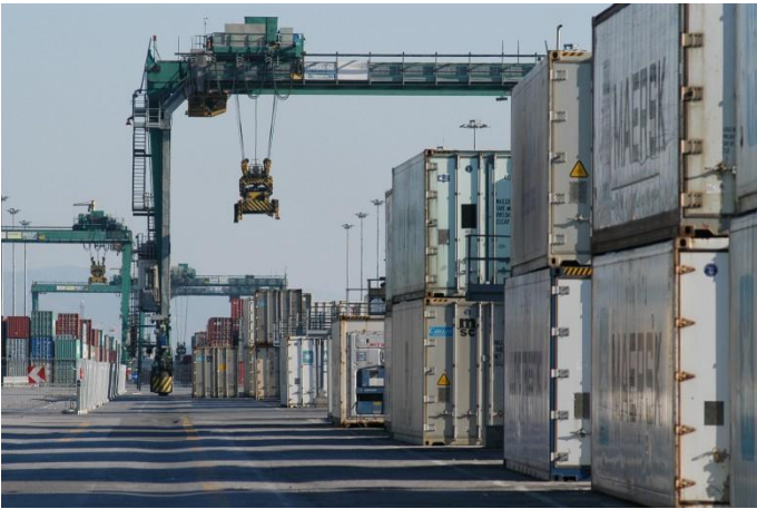
Figure 4. The Yard with the rubber-tired gantries and rail-mounted gantries
