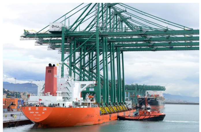
Figure 3. VTE’s quay gantry cranes - gooseneck type
