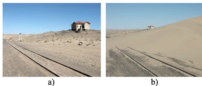
Fig. 3. Grasplatz railway station along the Aus to Lüderitz railway before (a) and after (b) sand dune encroaching (permission to reuse under a Creative Commons Attribution License; owner of the photos: Dierks, 2004 ).
