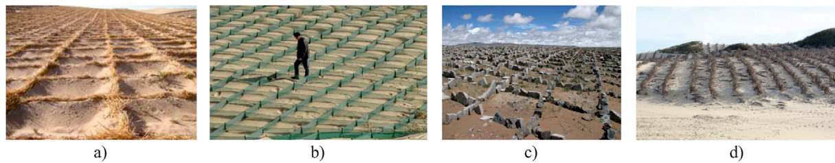
Fig. 14. Structured Hedge system: a) straw checkerboard (reprinted from: Guo et al., 2014, with the permission to reuse under a Creative Commons Attribution License), b) polyethylene-net checkerboard (reprinted from: Zhang et al., 2010a, with the permission from Elsevier), c) stones checkerboard (reprinted from: Zhang et al., 2010a, with the permission from Elsevier), d) array of line-like obstacles (reprinted from: Lima et al., 2017, with the permission to reuse under a Creative Commons Attribution License).
