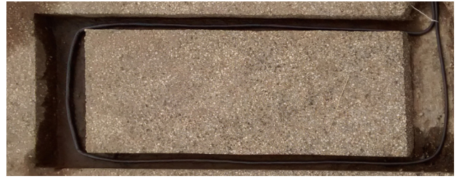
Fig. 7. Structure of the transmitter coil for system B during the embedding in the road surface.
