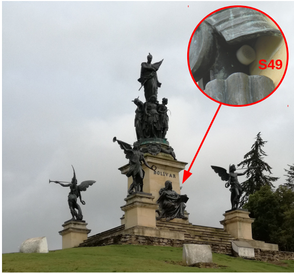
Fig. 4. Placement of the sensor node S49 on the Von Miller Monument (Ponte de Boyacá).
