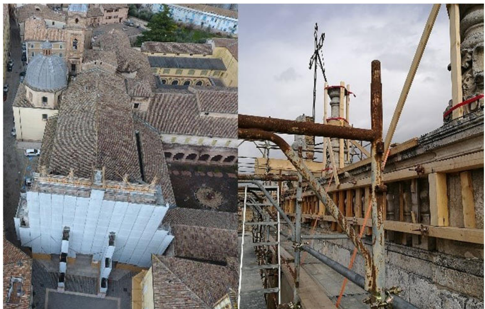
Fig. 5 Basilica di Tolentino. Provisional structures after the seismic events
