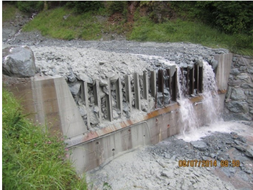
Fig. 4.1 Image recorded after the event on 11-07-2017 event in Saint-Vincent (AO), Italy. Also grains smaller than the outlets width of the sectional barrier clog and are retained behind the barrier. Courtesy of Valle d'Aosta Region.
