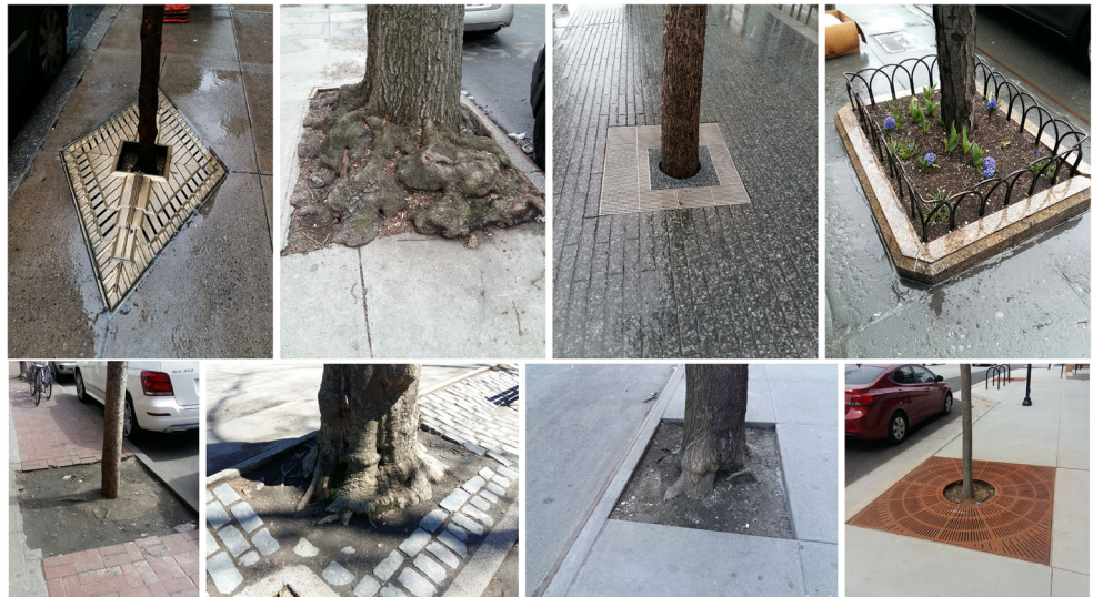
Fig. 1 Examples of bare soil extension and permeable/impervious configurations surrounding street tree installations. The last picture in row two refers to Chapel Hill (NC), others pictures refers to New York
