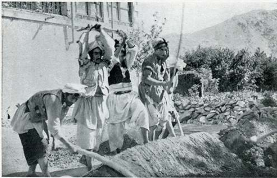
Figure 1b: Traditional Afghan building techniques: Afghan construction workers beating lime, brick dust, and vegetable fibers, to be employed as a substitute for concrete.
