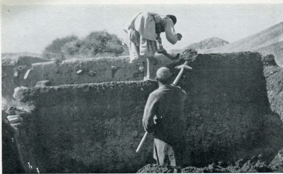
Figure 1a: Traditional Afghan building techniques: water, clay and straw, the materials used for the construction of walls.
