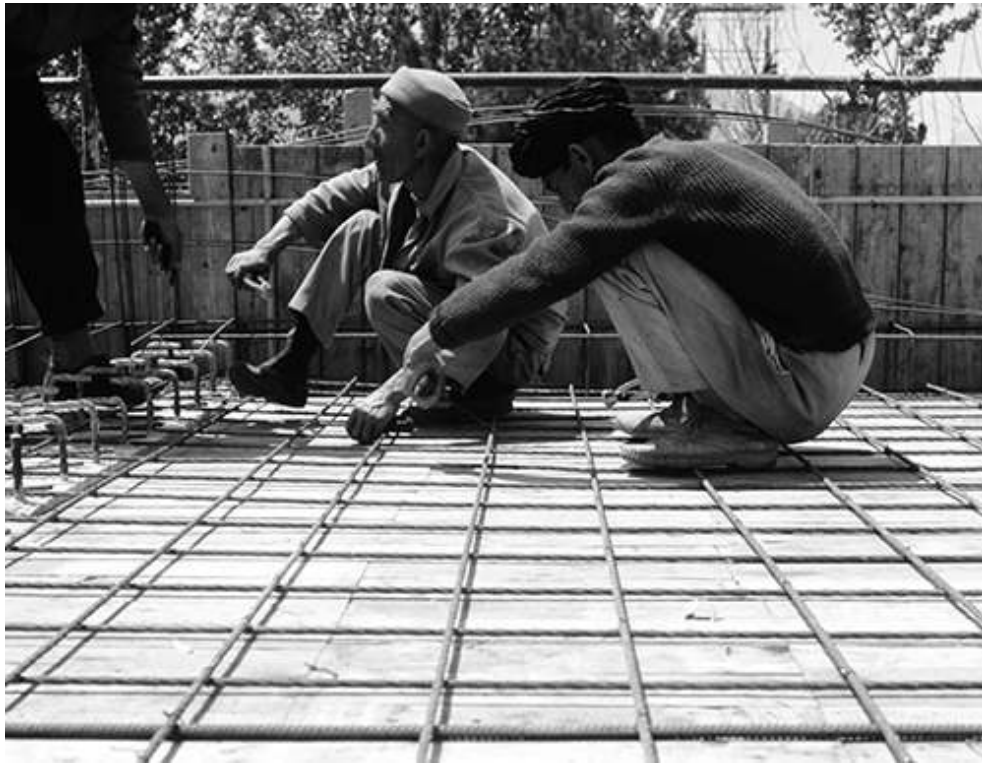
Figure 3: Afghan workers installing the reinforcing bars for the embassy's roof.
