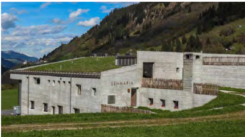
Caseificio alpino Sennaria a Disentis/Munster, CH, arch. Gion Caminada, 2010
