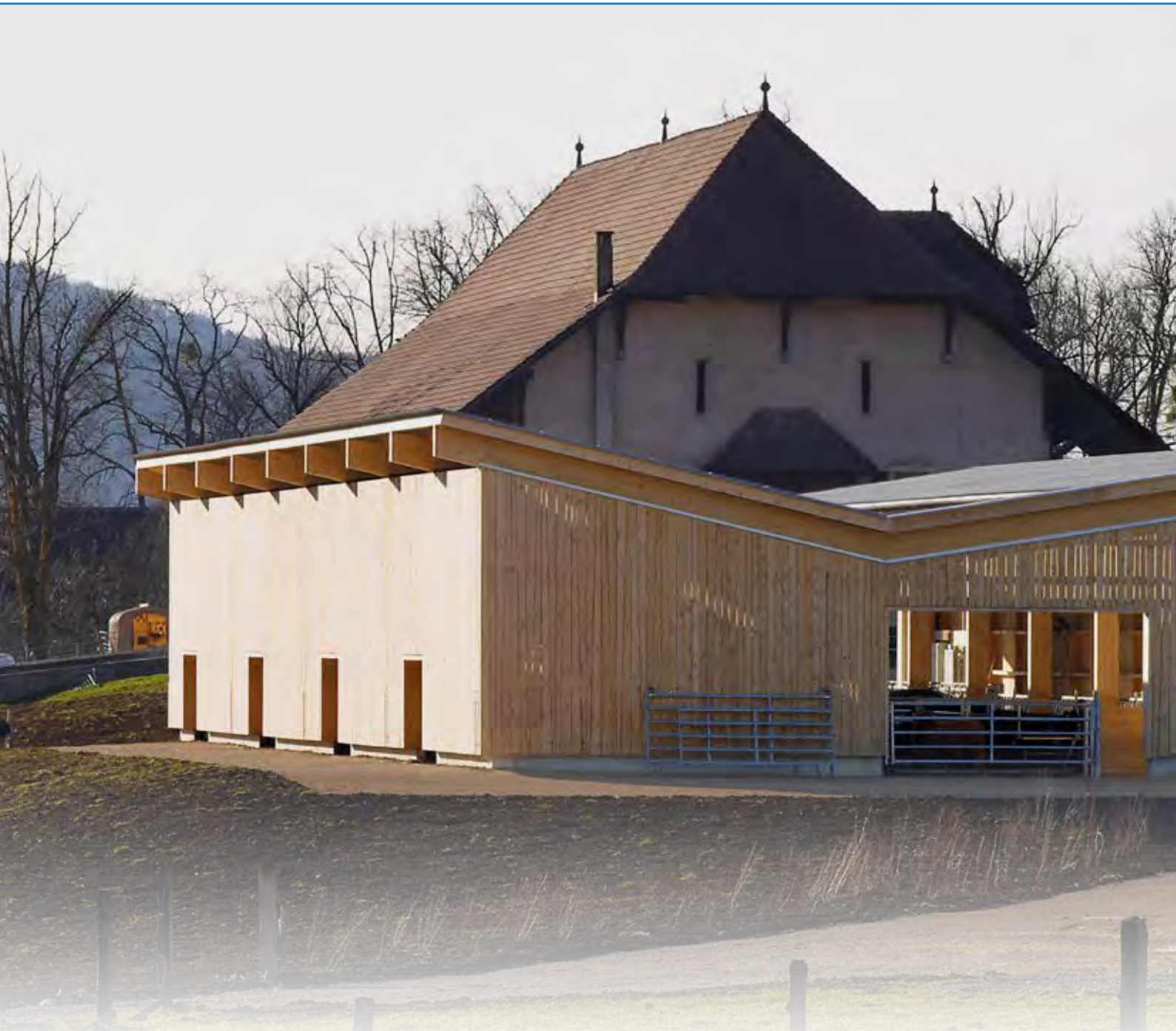
Stalla a Wildenstein, CH, arch. Kury Stahelin, 2013 (fonte www.staehelinarchitekten.ch )
