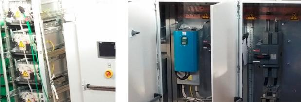
**Electric cabinet. Ultra Capacitors, operator panel and emergency red button, DC/DC converter and a manual switch.**
