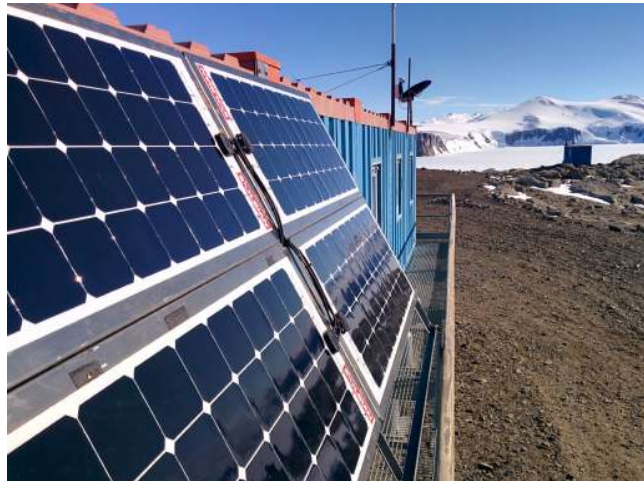
Fig. 4 Solar panels used as primary source of energy from the system.
