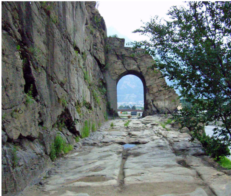
Figure 1: The Roman road to Gallia, near Donnas in Valle d'Aosta (Courtesy Lysippos, Wikipedia). Note the two grooves worn into the road by the passage of wheels.
