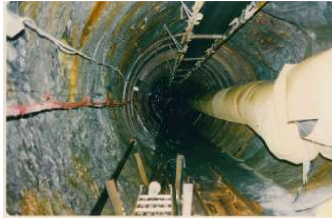
116 Figure 3. Hydropower tunnel in Northern Italy. Local damage and irregular profile at rib is due to spalling in 117 metamorphic rock mass and anisotropic state of stress, even if mechanised tunnelling with a full face open TBM has been 118 adopted. Suggested D = 0.7 . (Photo by C. Oggeri)
