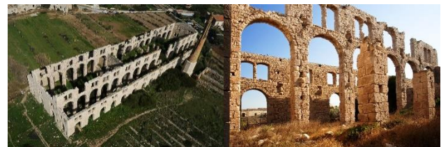
Figure 3. Fornace Penna in Scicli: view from a UAV image acquired for the test (left) and inaccessible inner space (right).
