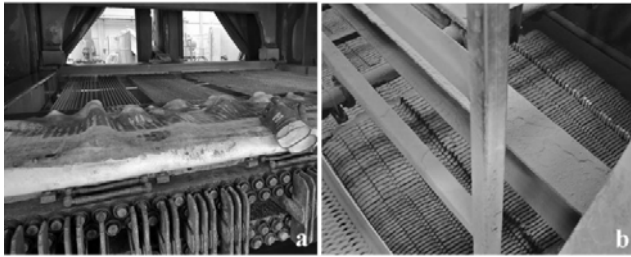
Fig. 3 Multi-blade technique. (a) Placement of blades in preparation to the sawing process; (b) Cutting of stone blocks into slabs
