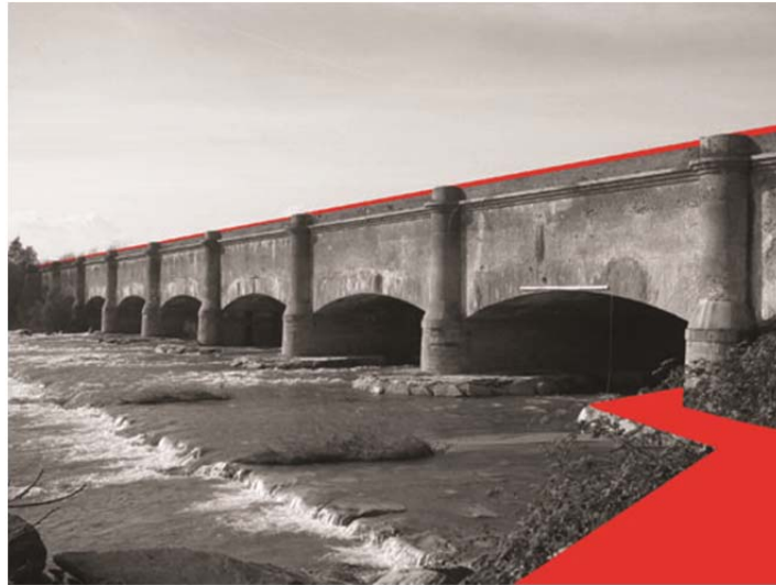
Figure 5. View of the cycle-route on a bridge-canal. Source: Ocelli, Palma and Sassone, 2012.
