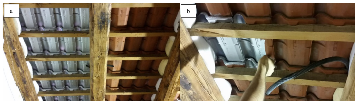
Fig. 3. (a) on the left (config B), on the right (config. A); (b) Low-E treatment by paint brush coating
