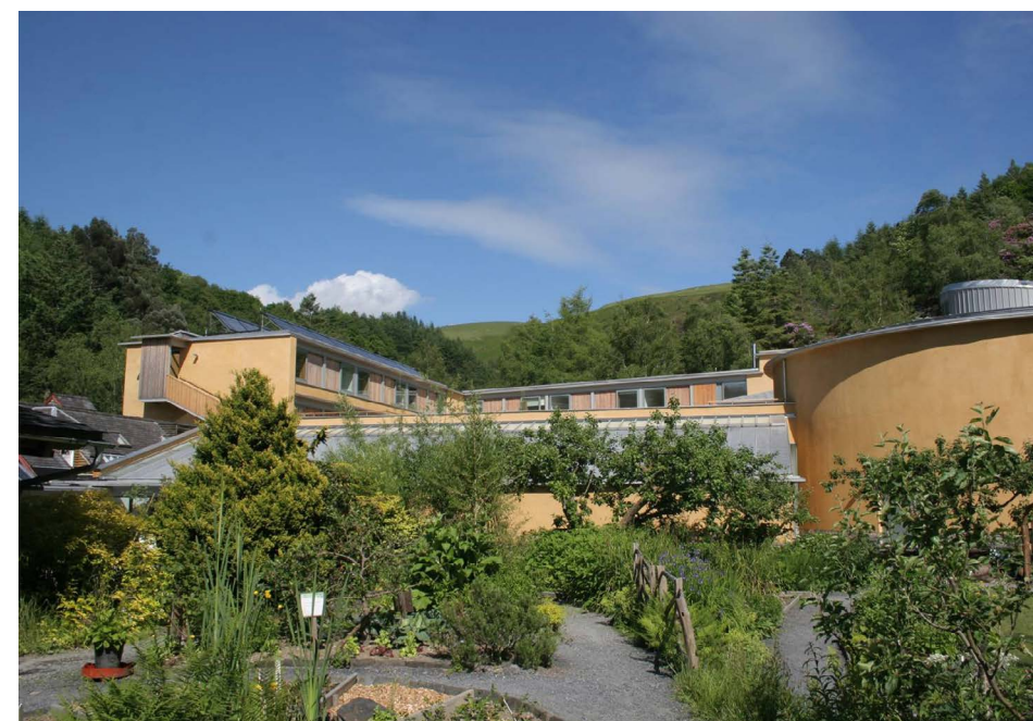
Fig. 8 Welsh Institute of Sustainable Education (WISE), al Centre for Alternative Technology, Machynlleth (Powys).
