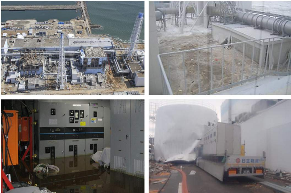
Figure 8.28 Photographs of the Fukushima nuclear power plant after the 2011 Tōhoku earthquake and tsunami.
