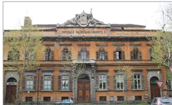
Figure 7.1 Umberto I, Mauriziano hospital in Turin.
