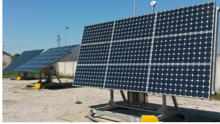
Figure 3. Example of misalignment between the plant A_{is} (right-side of the picture) and the plants D_{is} and E_{is} (left-part of the picture).
