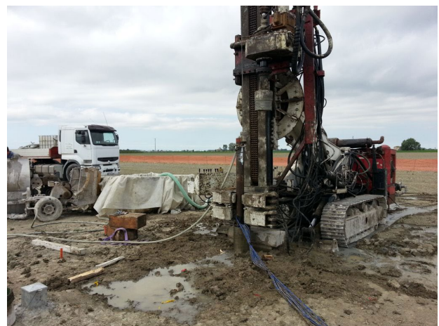
Figure 6. Installation of the instrumented micropile.
