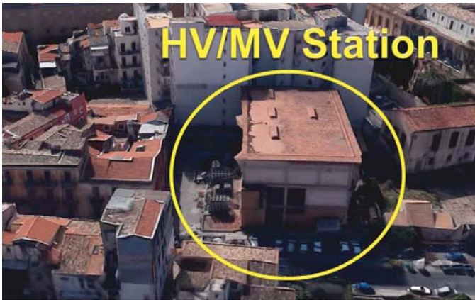
Fig. 1. Example of HV/MV station integrated in an urban area with residential building in the neighborhood.
