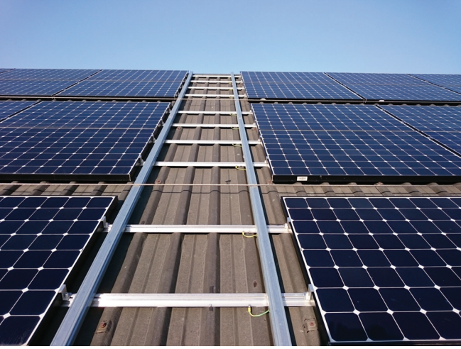
Fig. 3. PV modules, aluminum frameworks and bonding conductors.
