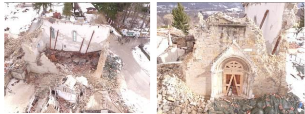
Figure 5. Oblique image of the Sant'Agostino Church; the top of the bell tower and the collapse after the Norcia earthquake; the structure after the January seismic events
