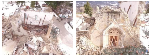
Figure 5. Oblique image of the Sant'Agostino Church; the top of the bell tower and the collapse after the Norcia earthquake; the structure after the January seismic events
