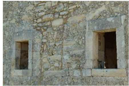
Fig. 10- Tower-house in Giannoudion, exterior North façade, detail (Emma Maglio, 2014).
