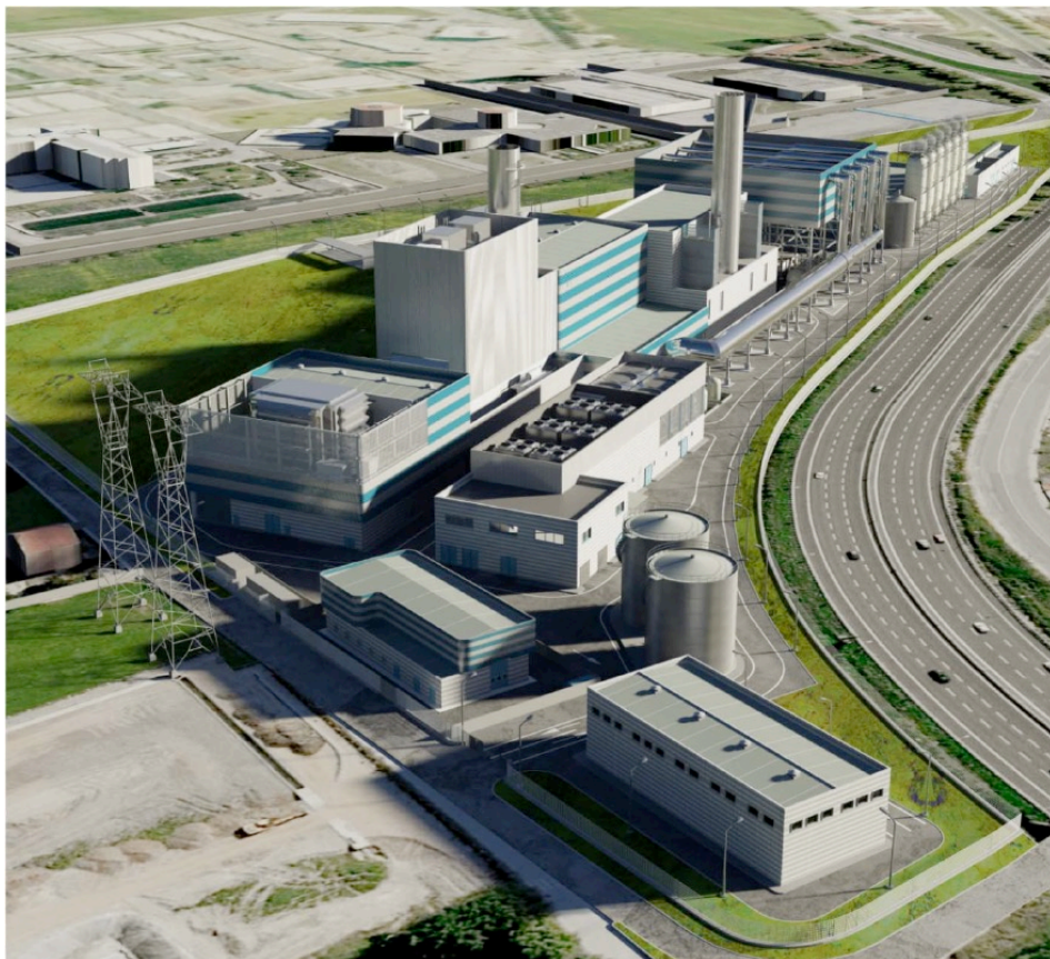
Figure 3.6. Image of Torino Nord plant. (source: Iren Energia, 2014b)
