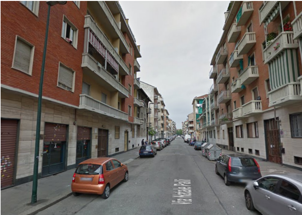
Figure 3.3. Representative picture of the buildings interested by the potential DH network extension (source: www.google.it/maps ).
