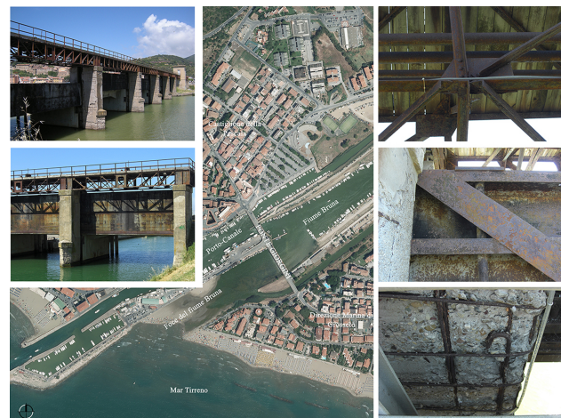
Figure 1. The Giorgini Bridge
