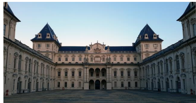
Figure 1. View of the Valentino Castle courtyard
