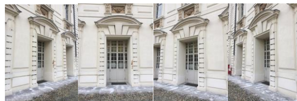
Figure 3. Part of a dataset acquired by a Canon 600D with a 18 mm (shooting distance= 3 m; GSD= 0.7 cm )
