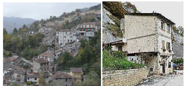
Figure 1. Pescara del Tronto perched village, in Arquata del Tronto, AP, October 2016 (left). The object of focus: a stand-alone damaged building (right).
