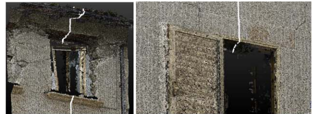
Figure 18. Section (4) on terrestrial photogrammetric model
