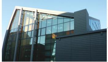
tensioned beams in laminated wood that is hinged to a single reinforced concrete pillar and braced by the metal cylinder of the lift shaft. The exterior side facing the street is entirely glazed, thus making the climbers visible day and night. The roofing and part of the facades are coated with grey zinc-titanium which evokes the colours of the mountains, while the interior space
